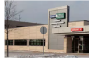
Froedtert Community Hospital - Oak Creek 7901 S. 6 th St Oak Creek, WI 53154
